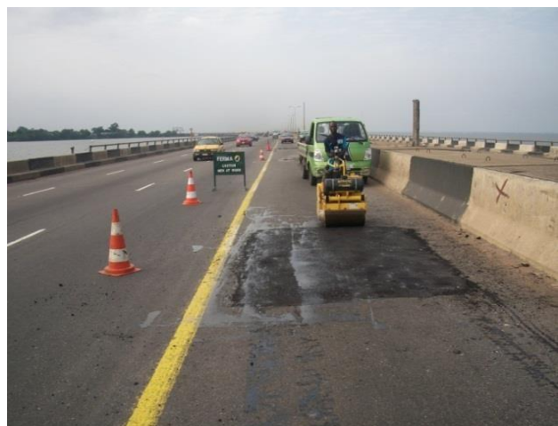
PATCHING OF POTHOLE WITH ASPHALT ON THIRD MAINLAND BRIDGE, LAGOS
